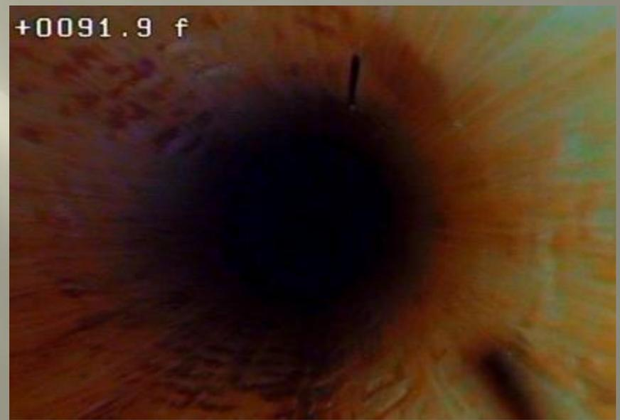
Due to our pumping, the water level had dropped about 3 feet. But as soon as the camera went underwater, everyone was shocked to see how clear the water was. Immediately we noticed we could see the cut perforations in the PVC casing.
