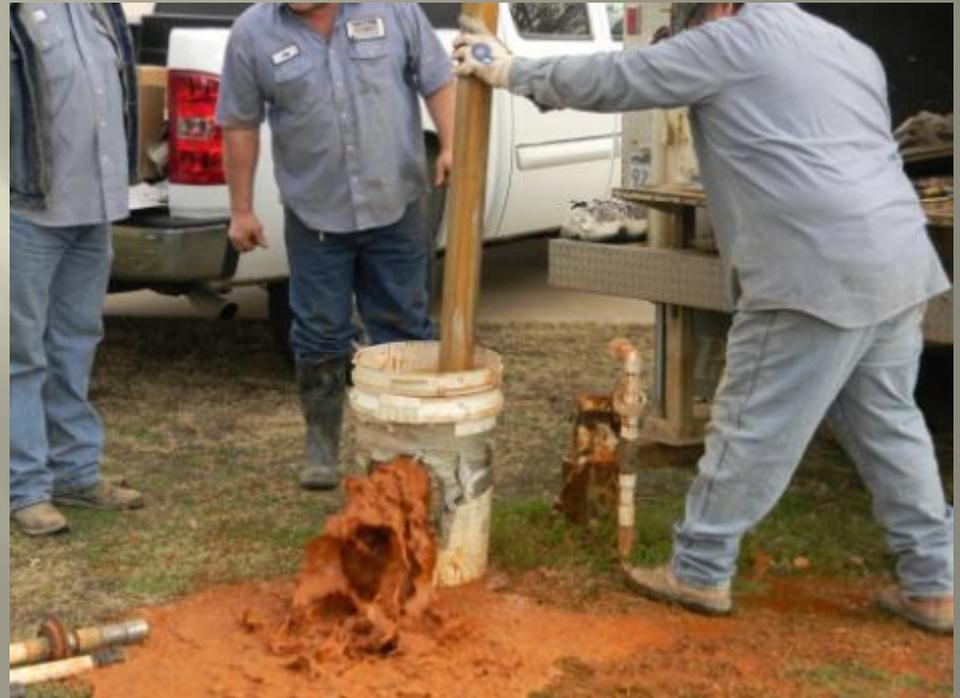
After the video, we bailed the hole about 12 times (to remove as much of the big pieces knocked loose by pulling the pump and the brushes as we could).
