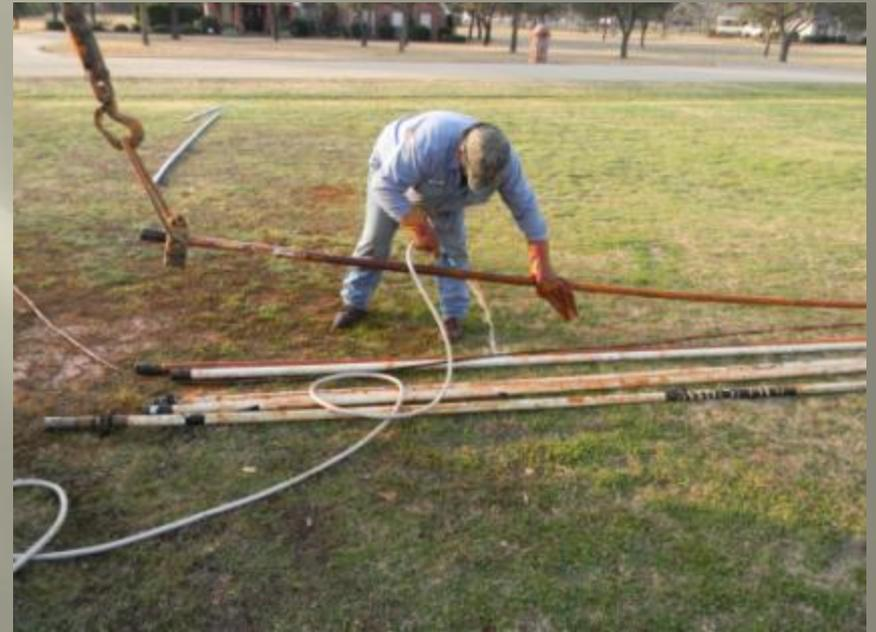
We arrived the next morning and started to put the pump and drop pipe back in. We rinsed off as much of the IRB from them as possible before we put them back in the hole.
