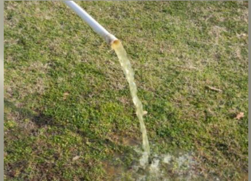
We weren't sure how long we were going to be able to pump because a thunderstorm was approaching. So we decided to pump for 20 minutes, then let the hole recover for 10 minutes, and to keep this up for 2 hours. At first when we did this, we would get a charge of reddish-brown water each new time we cycled on the pump. But eventually this was lessened, and eventually we didn't get any more charges of brown color.
