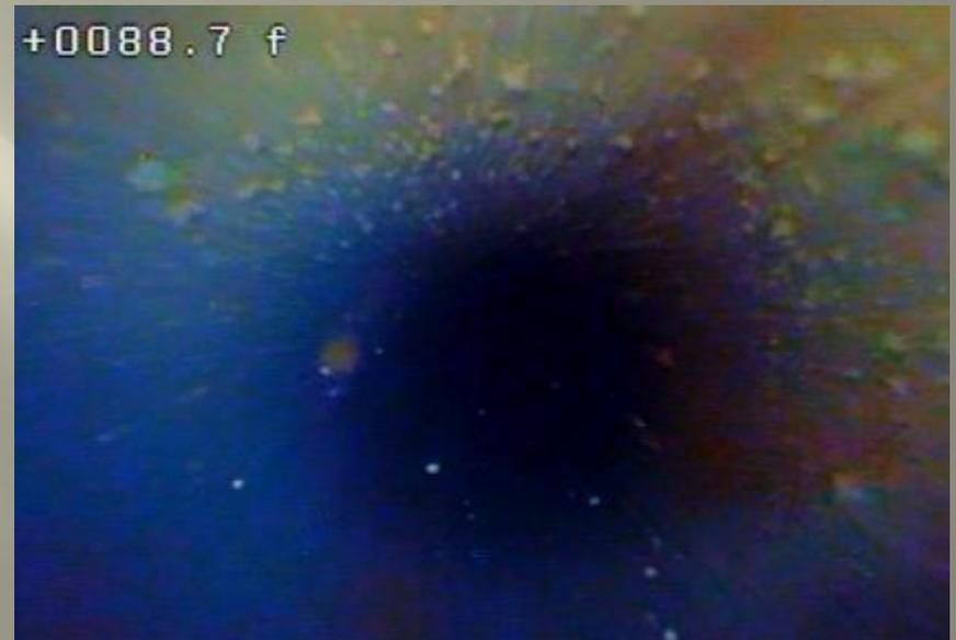
The pipe above the static water line was stained from the IRB, and as soon as the camera went under water, large globules of iron bio film were so prevalent it was hard to find a spot where a picture could represent what we were seeing.
