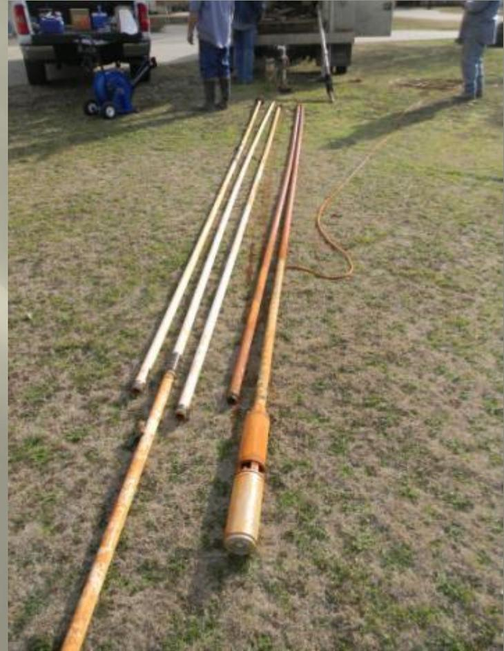
We were going to use the bailer as a block to knock off debris before we brushed, but we figured the pump already did that when we pulled it out of the 4" hole. Here you can see how bad the iron problem is on the pump and the drop pipe.
