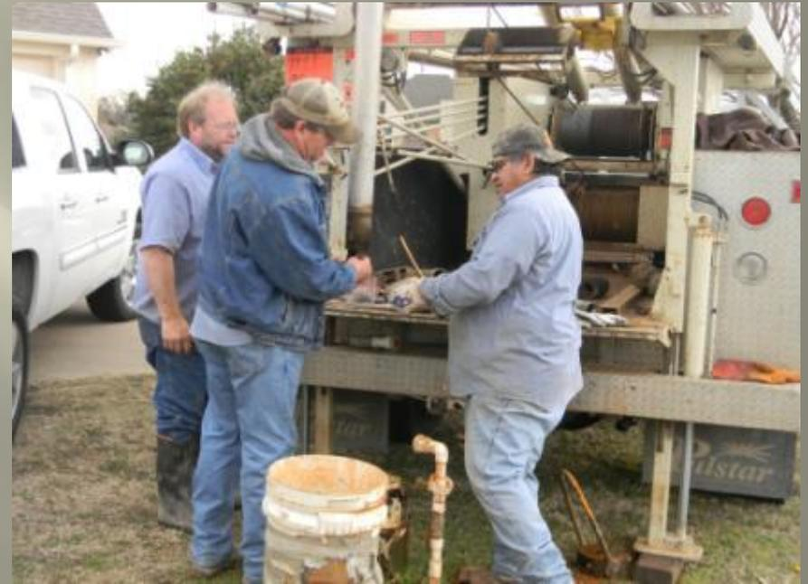
We rinsed the column down real well, then sealed off the bottom of the bailer and ran it up and down the column for 30 minutes to act as a surge block to push the Ultra C through the slots and into the gravel pack.
