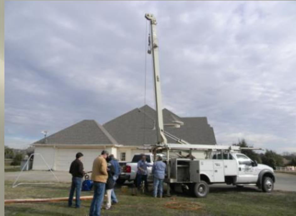
After pulling the pump, we ran a 4" brush in the hole about 30 minutes. We then set up the camera and made a visual inspection.
